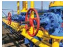
**Distribution pipelines** deliver natural gas directly to customers and, like **transmission pipelines**, can have an impact on people and property if damaged by digging or excavating. The majority of underground **distribution pipelines** are generally **not** marked aboveground, so it is critical to call **811** to have the lines located **before** you begin any digging, gardening or excavating. This service is **free**.
