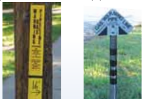
Examples of transmission pipeline markers.
