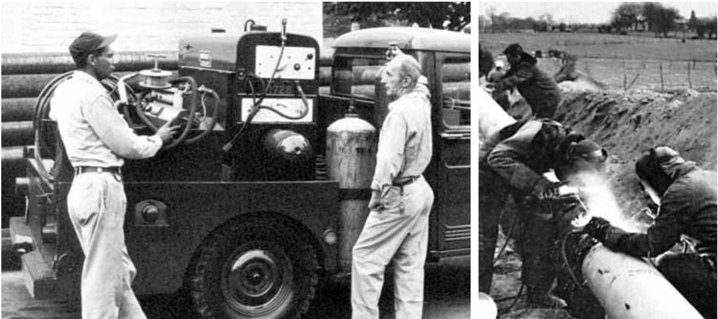
*New dual purpose welding equipment (left) was state of the art for its time, and helped with major expansion projects, such as the installation of this 12-inch main in Virginia (right).*
